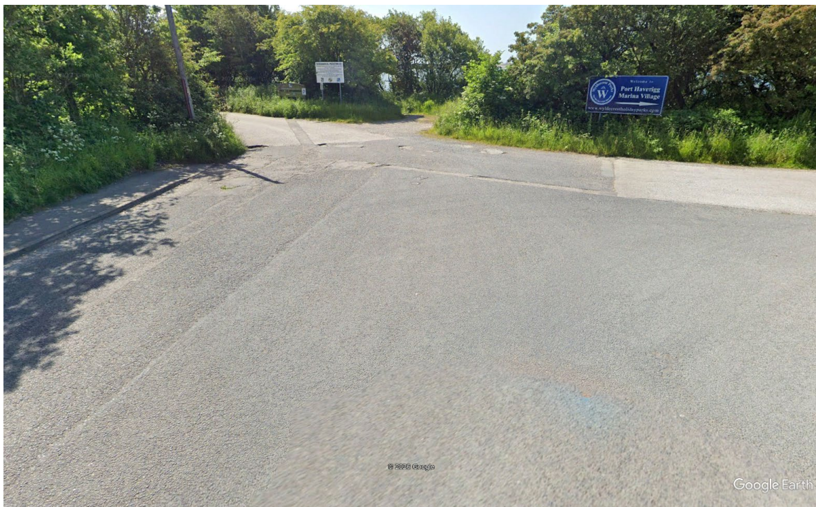
Figure 2. View of the affected junction, showing the tarmac carriageway and hardstanding within the application section. Source: Google Earth image supplied for the assessment.
